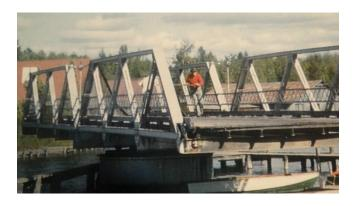
In 1905 the one hundred room Pere Marquette Hotel was opened on the shore of Torch Lake north of Clam River. Concern that a new bridge was needed to handle all the traffic, a steel bridge was constructed over Clam River by the Huston and Cleveland Bridge Company. This was a hand-operated swing bridge.
